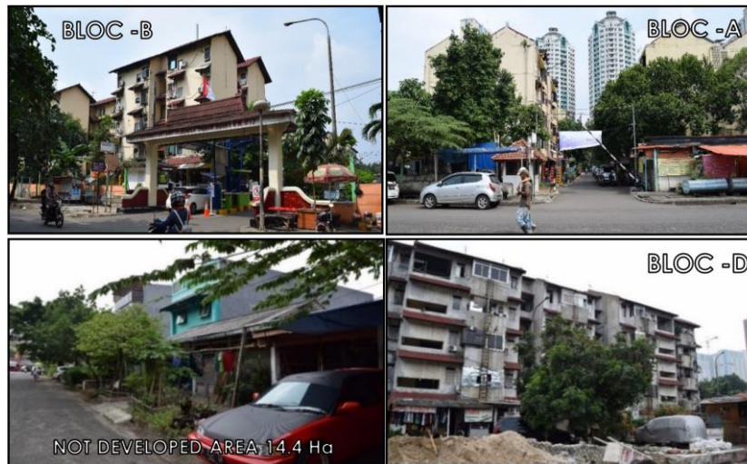
Figure 4. Condition of Kemayoran Flat Complex in high density and worsening environment.
