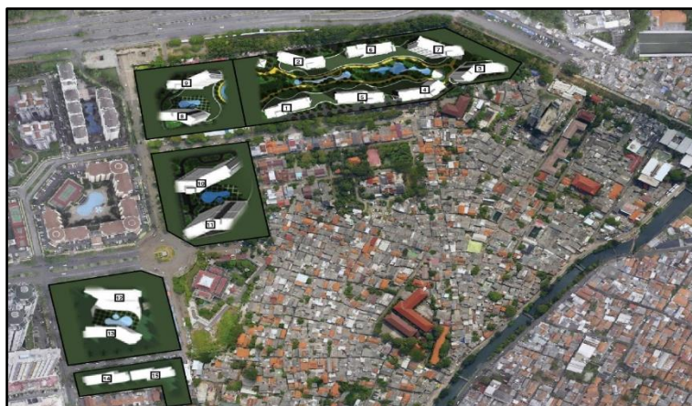
Figure 14. Final Completion of Renewal - Kemayoran Apartment Complex.
