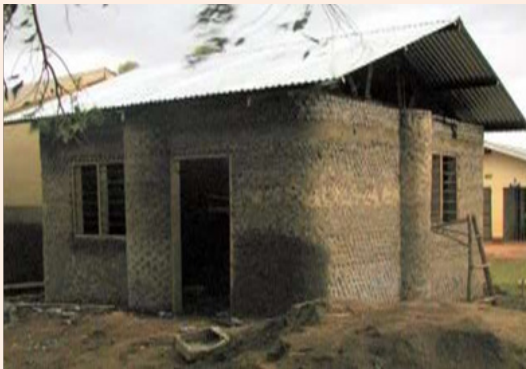
Figure 3: First bottle house construction.
