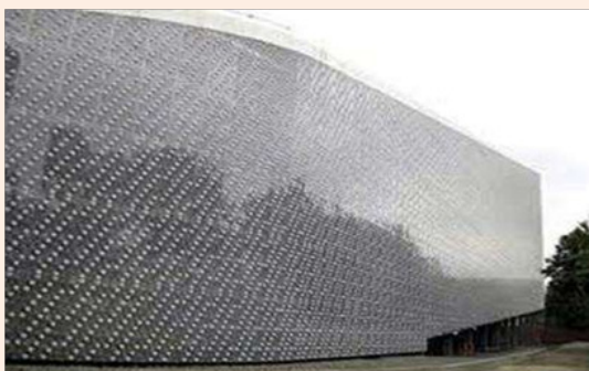
Figure 4: Eco-ARK built for taipei's.
