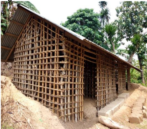
Fig. 3b: Corrugated Zinc roof on bamboo house
