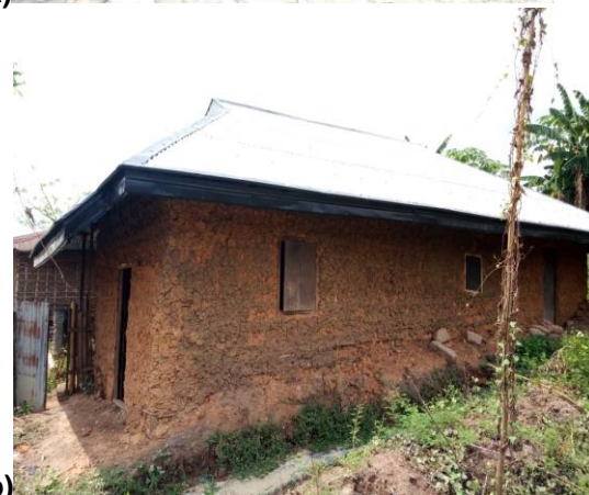
Figure 2a and b: Bamboo buildings finished with rammed mud mortar
