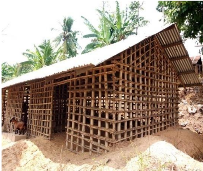
Fig. 1: Building walls constructed with bamboo
