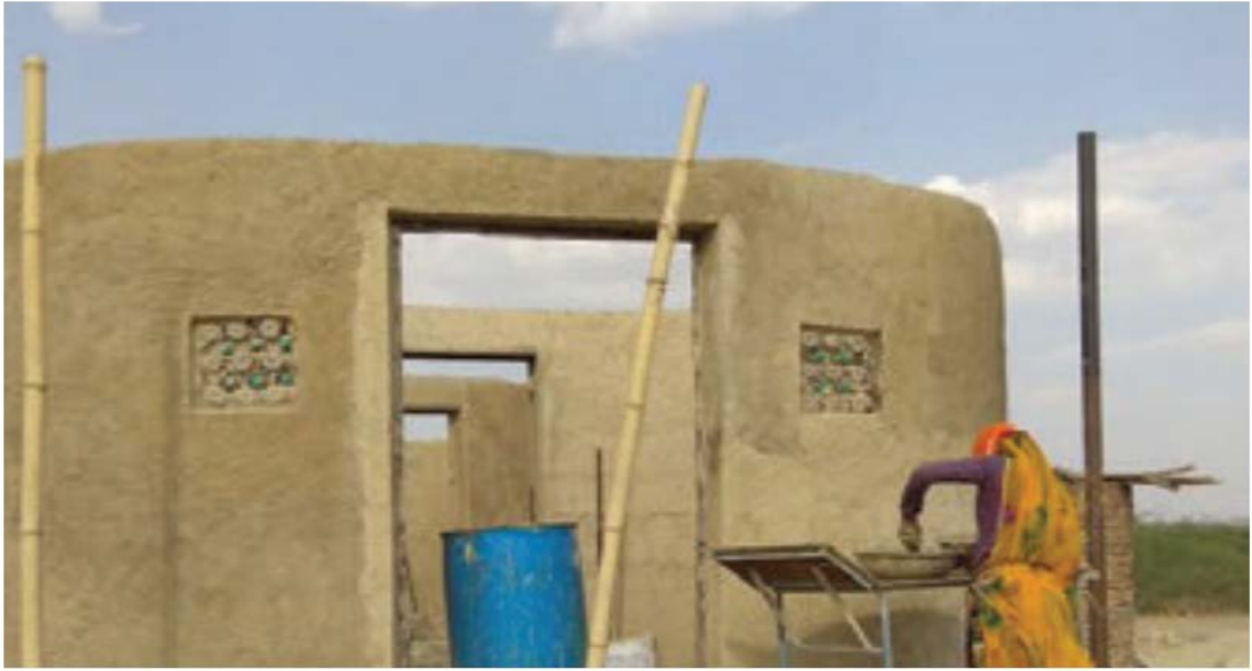
Figure 10. The completed Structure. Source: (Plastindia Foundation, 2019)
