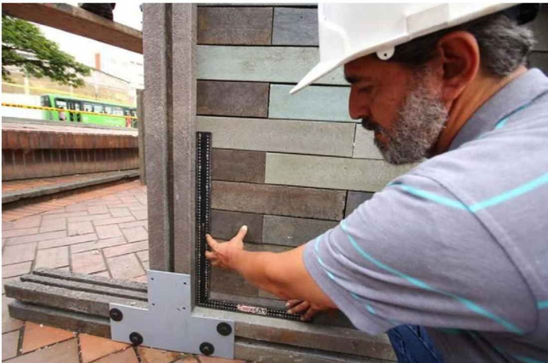
Figure 4. Building a House out of Recycled Plastic. Source: (ConceptosPlasticos, 2019)
