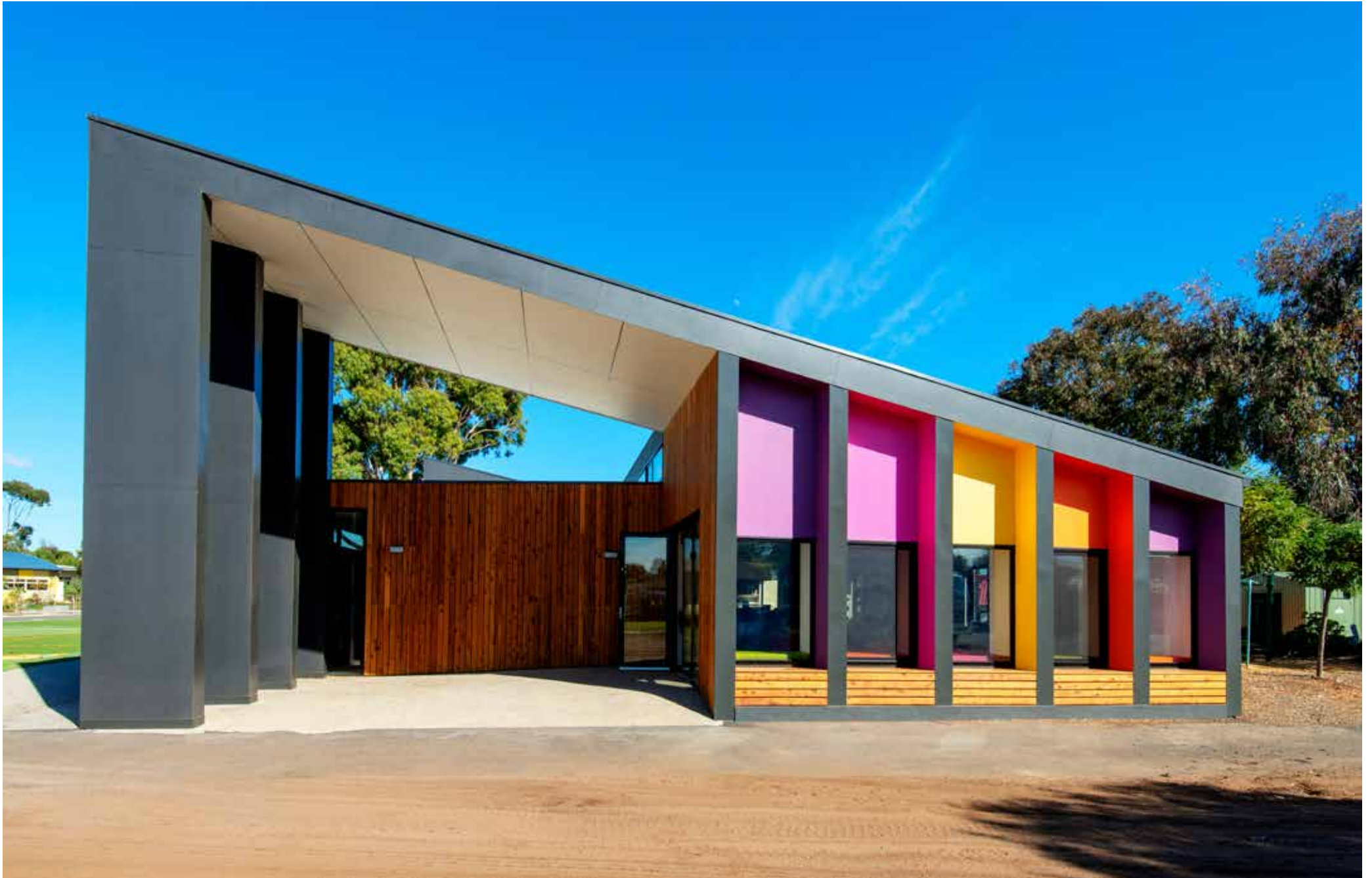
Picture: Altona Primary School, Victorian School Building Authority with ARKit and Sensum Group
