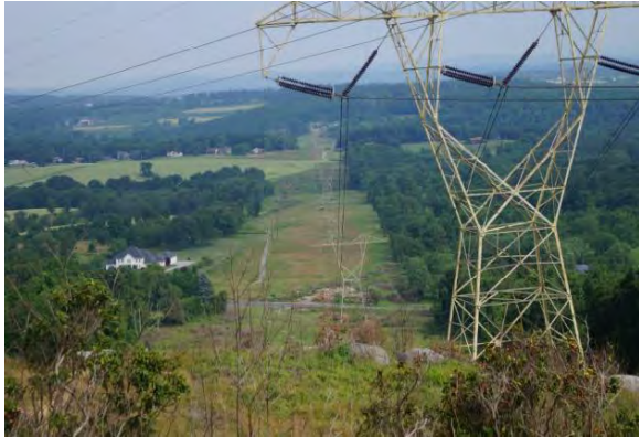
Figure 10: High Voltage Electrical Corridor in Rocky Ridge County Park (YCPC Photo).
