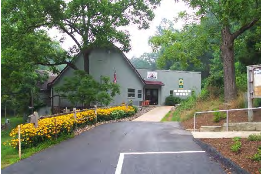
Figure 14: The Nature Center at Nixon County Park
