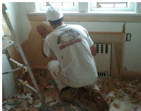
Lead Based Paint Abatement, YCPC photo
