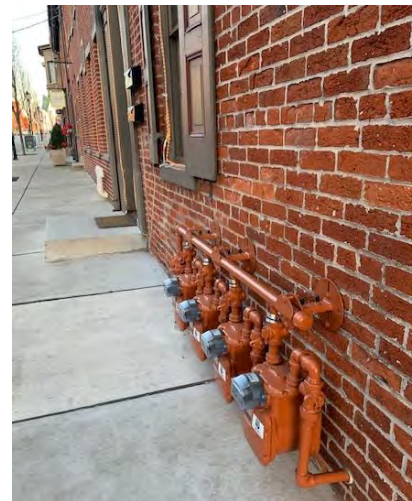
Figure 15: New Gas Meters in a Historic York City Neighborhood (YCCP)
