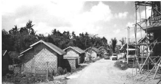
Figure 1. Dalung Permai – private housing project. Source: Acwin (2009).
