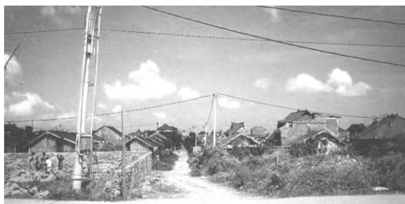
Figure 2. Road condition in Dalung Permai – private housing project. Source: Acwin (2009).
