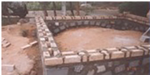
Fig. 4. Rattrap bond brick masonry
