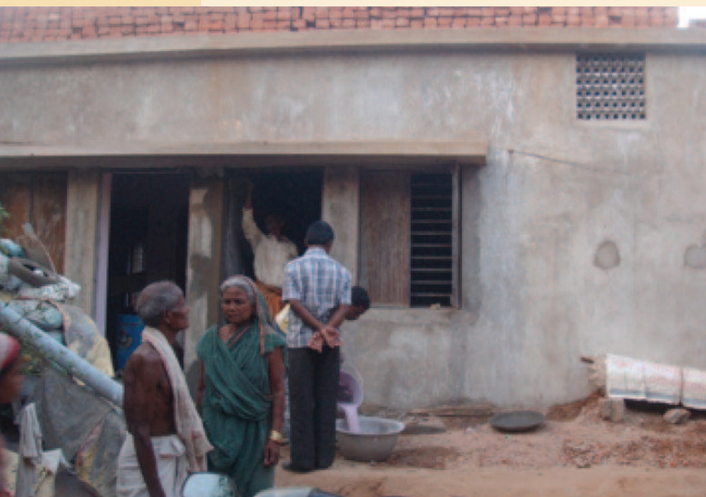
Picture 2 : A house under construction in Bhubaneswar.
