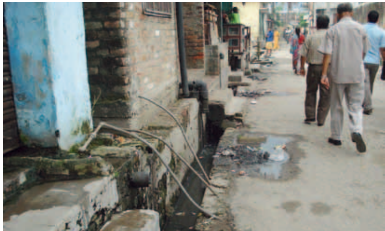
Photo7k: Open sewer in front of houses © UN-HABITAT
