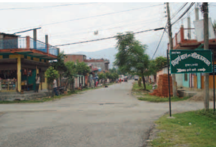
Photo7n: Newly black topped road in Butwal © UN-HABITAT
