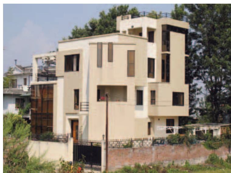
Photo7b: A lavish residential bungalow with poor infrastructure © UN-HABITAT
