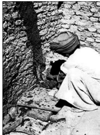
4. Starting the Inclined Course
