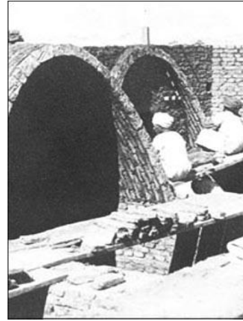
11. Building arch after arch
