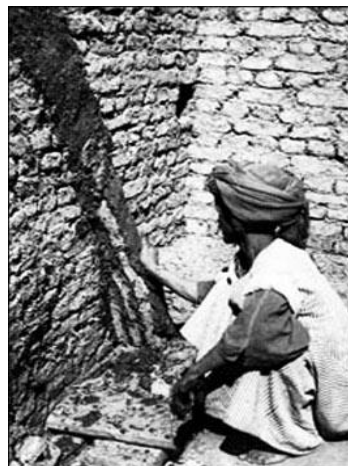
7. Applying some mortar
