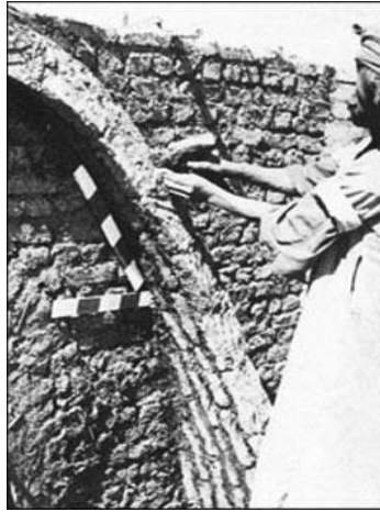
10. The first arch is completed
