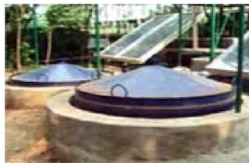
Figure 14: Biogas Unit at BARC
