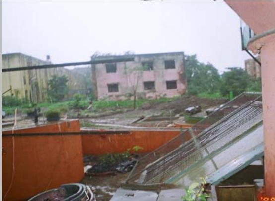
Figure 15 Solar Panels at the Biogas plant used for energy generation
