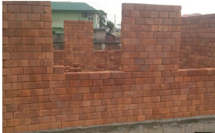
Figure 4. Dry-stacking of LIBs without mortar
