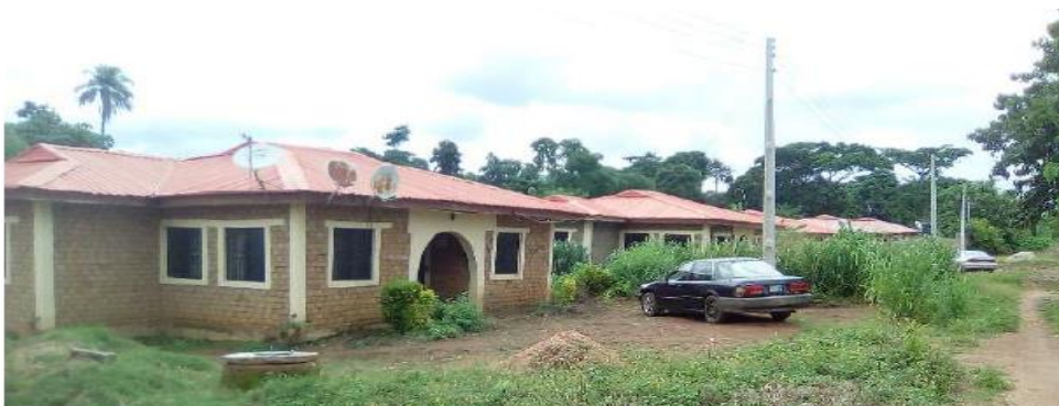
Figure 7. Pictorial view of Olusegun Obasanjo Housing Estate, Ado-Ekiti, Nigeria Source: Oyebamiji [30].
