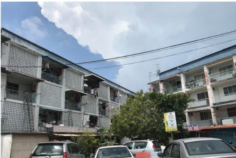
Figure 2. People's Court: Blocs C and D. Notes: Copyright © Woo KH (2022)
