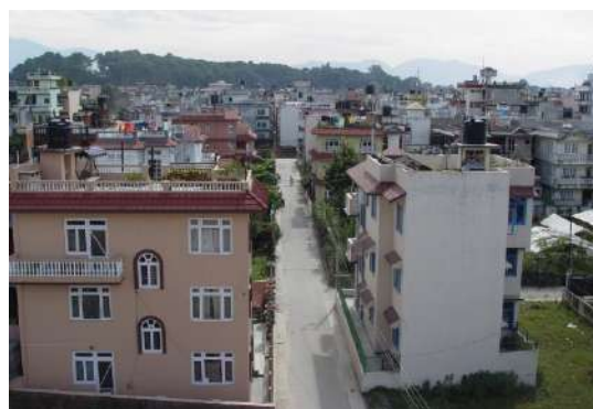
Residential development in Gongabu Land Pooling Project area (Photo: Sunil B. Shrestha)
