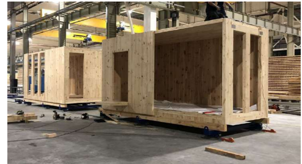
CLT modules have been produced on the plant in Korosten', Zhytomyr obl
