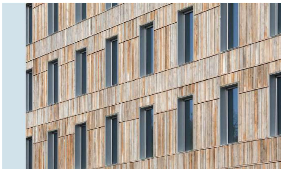
Creative wooden facade from reclaimed wood The Botanical Institute building of the University of Liège
