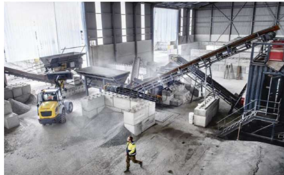
SmartCrusher installation, NL
