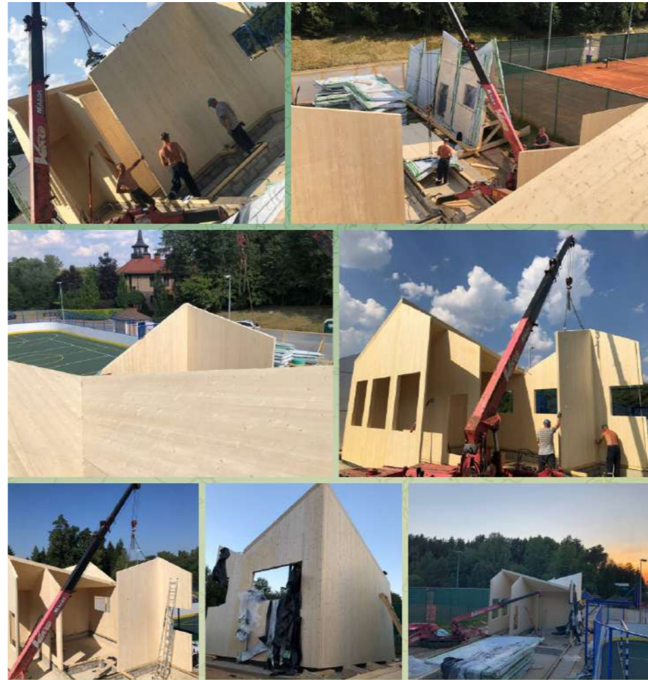
Source: private practice of Andrii Bidakov, engineer, expert in wooden constructions
