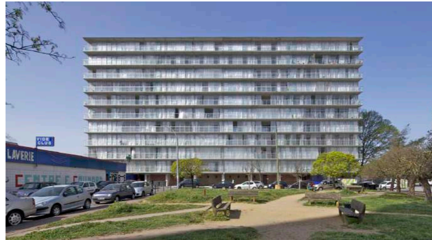
New facade. Soucre: Lacanton Vassal
