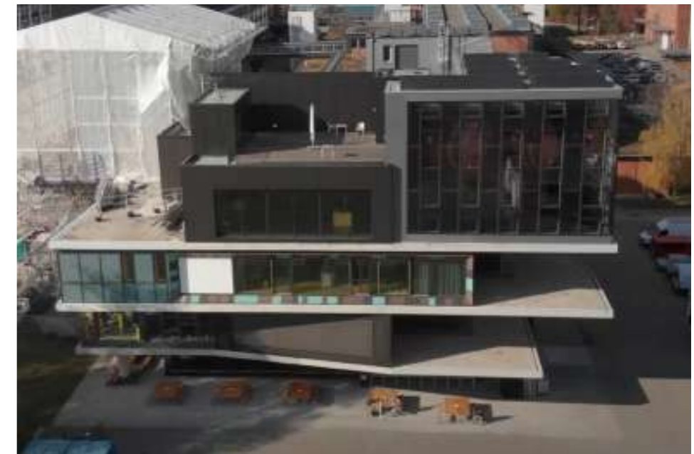
NEST building Source: EMPA youtube channel
