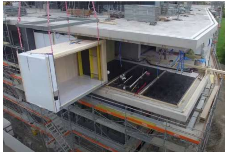
Installing a prefabricated module onto the concrete structure Source: EMPA
