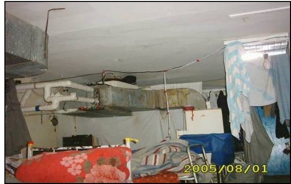
Figure 11. Using Service Rooms as Accommodation
