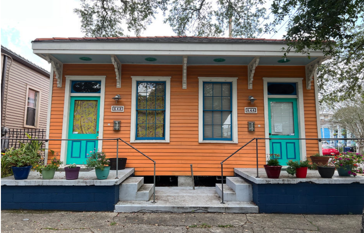
Figure 8. A duplex on a relatively small 2,500 square foot lot in New Orleans, Louisiana DMC Researcher Photo
