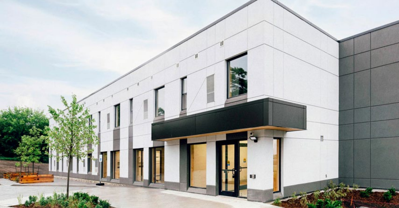
Multi-Unit Residential East Gwillimbury Passage House. Photo provided by Element5.
