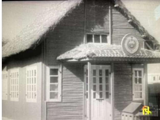
„A forest house of bamboo (06:42min).” The bamboo was previously treated so that it is protected against fire and vermin. Still from the film Modest Homes (1954).
