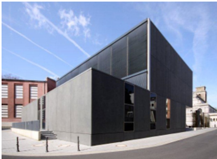
Fig. 15 TRC facades with AR glass Textiles at RWTH Aachen University [65]
