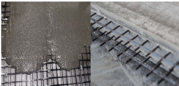
Fig. 1 Textile reinforced concrete casting process and hardened component [7]
