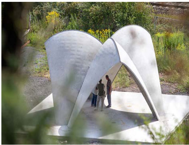
Fig. 12 TRC shell elements with six cast elements [60]
