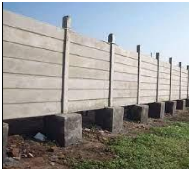
Figure 18: Precast RCC wall.
