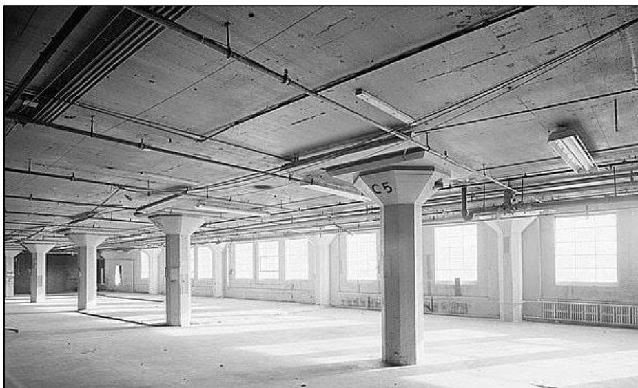
Figure 6: Flat slab system.
