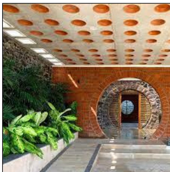
Figure 4: Filler slab system.
