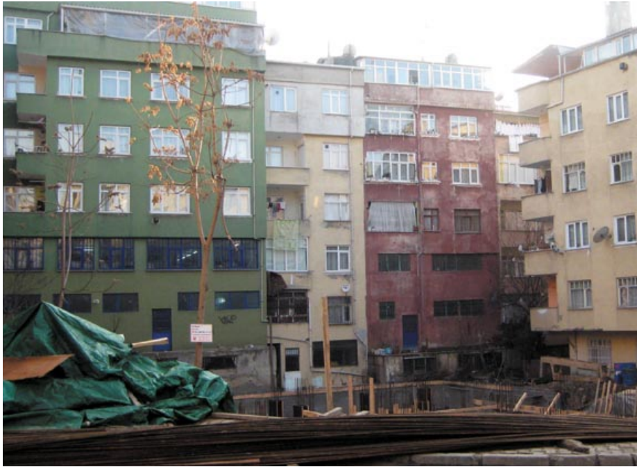
Construction site surrounded by multi-storey buildings
