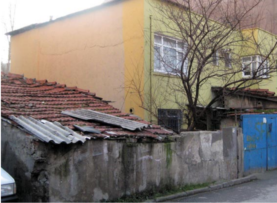
Buildings with added rooms
