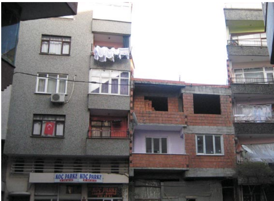
Adding another storey
