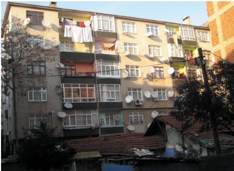
Six-storey buildings behind Gecekondu
