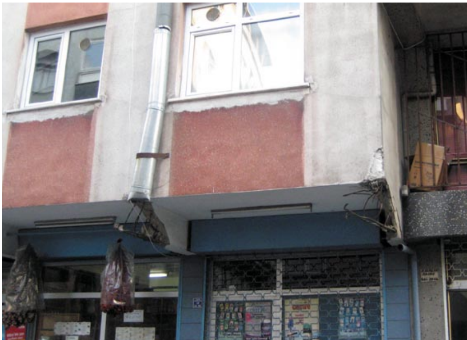
Exposed rebar
