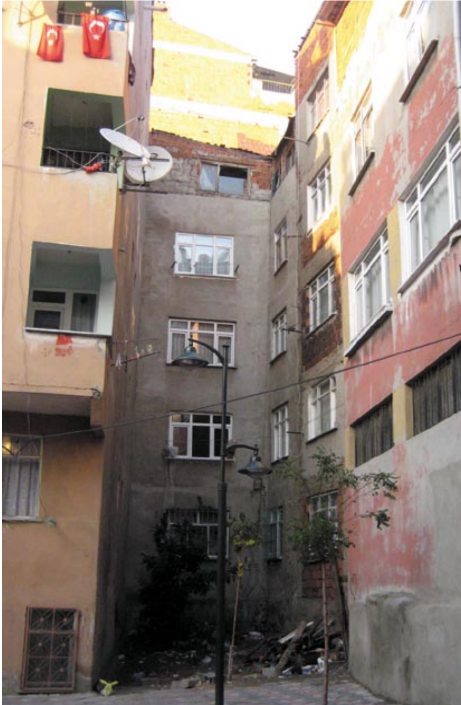
Yard between buildings with trash
