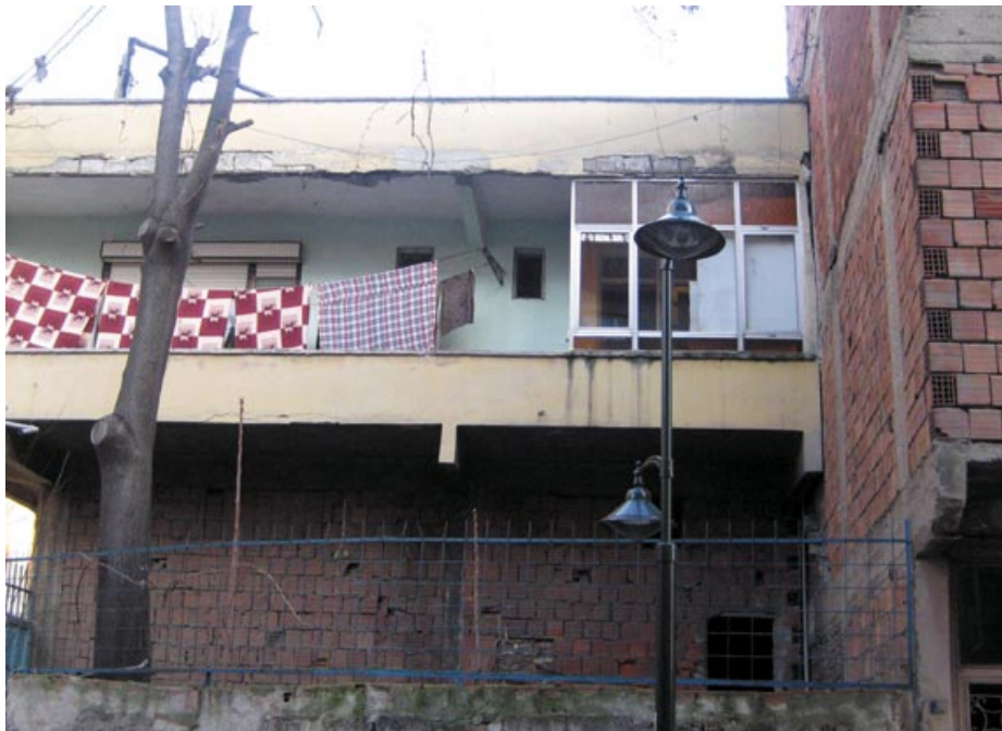
Complete second floor, incomplete first floor
