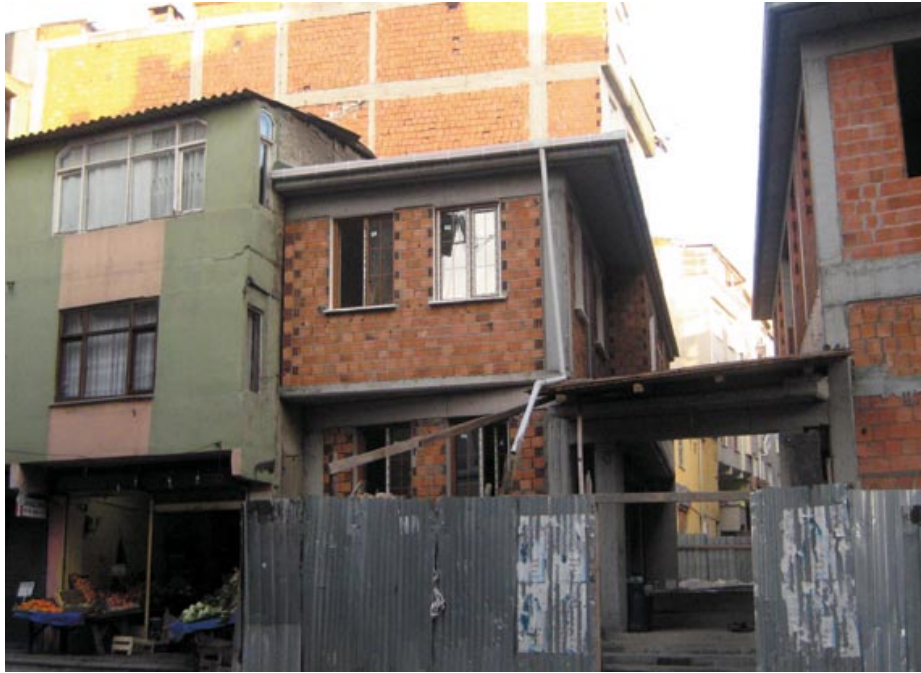
Constructing a two-storey building
