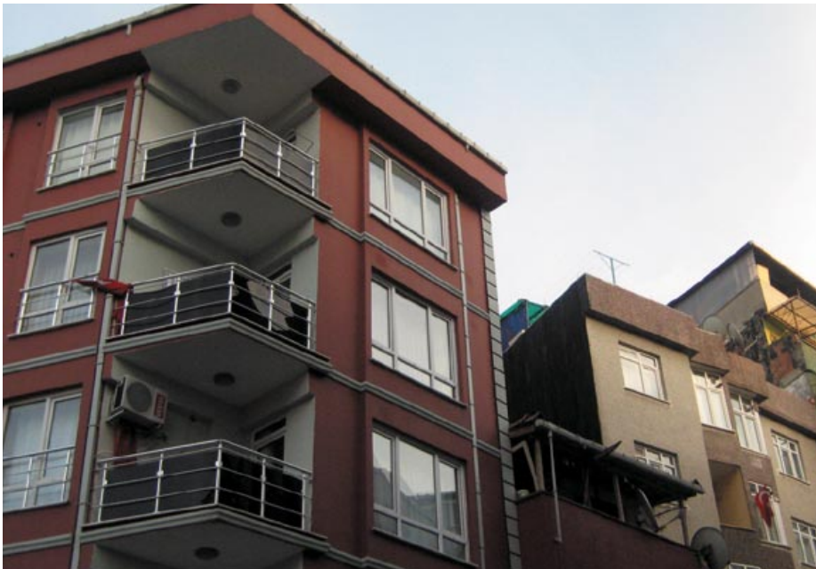
New construction (left) next to older buildings
