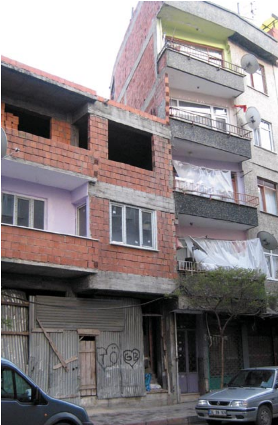
Ongoing construction between buildings
