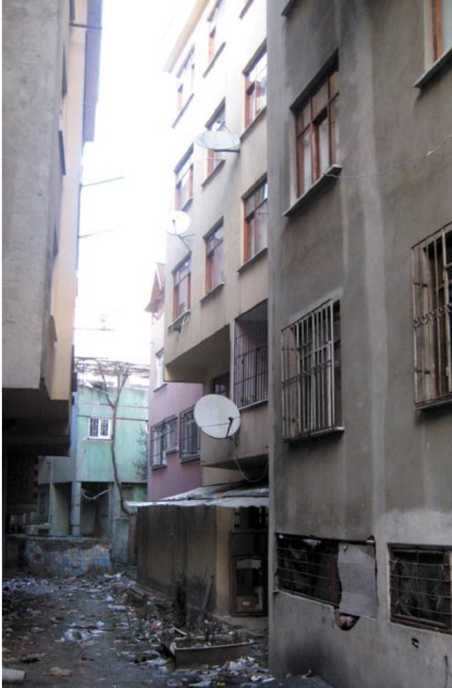
Trash between buildings
