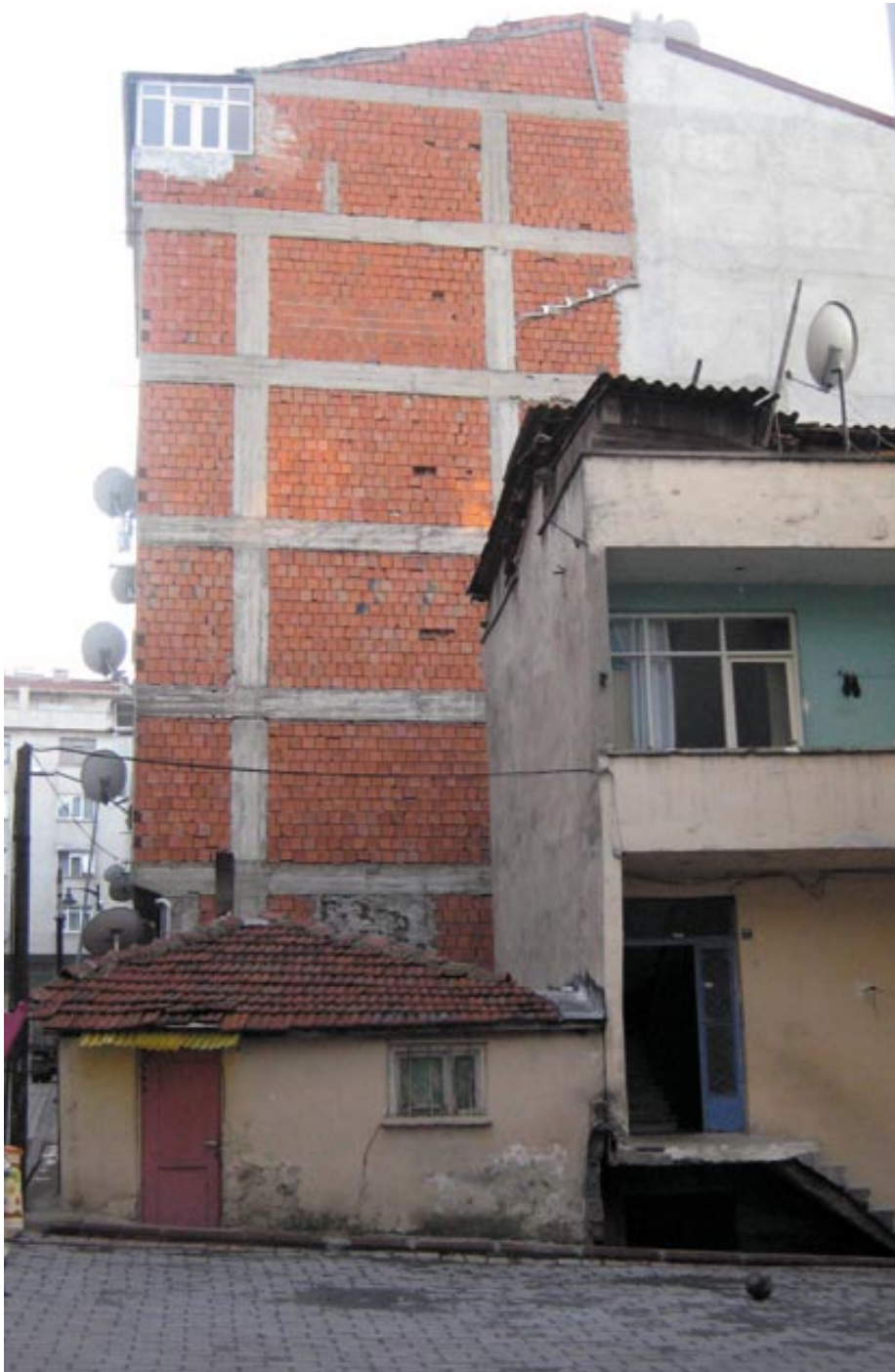
Half painted brick wall
