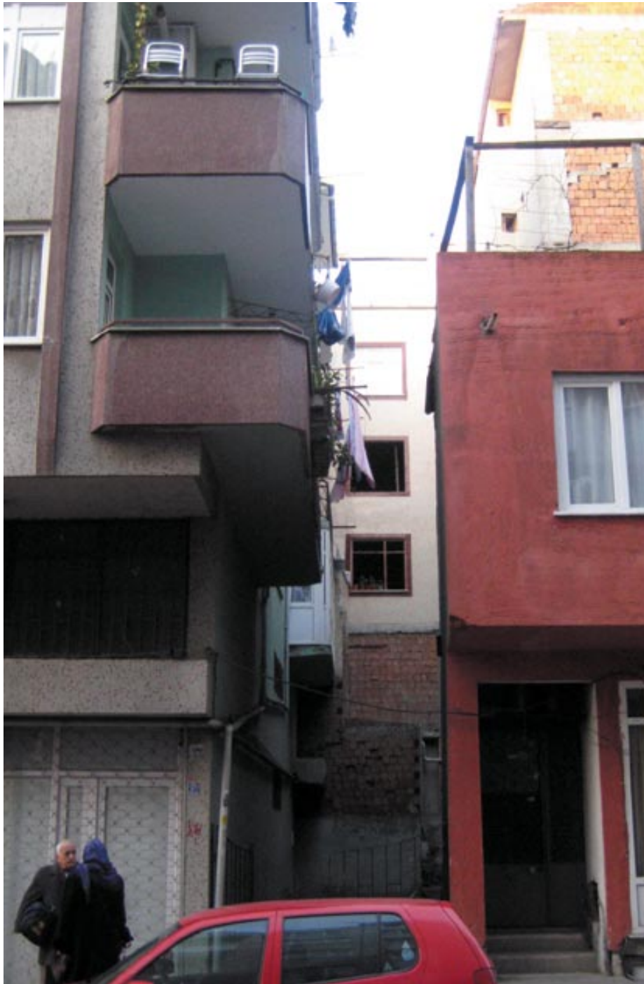
Closely spaced buildings
