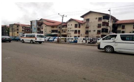
Figure 2: Block of Flats at Aggrey Road, A Low-cost Housing Estate
