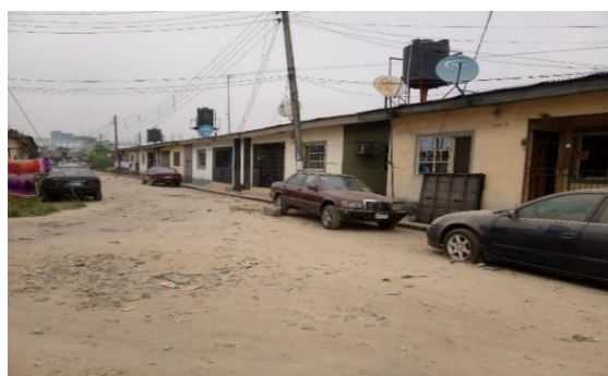
Figure 4: Semi-Detached Bungalows at Maine Base Low-cost Housing Estate
