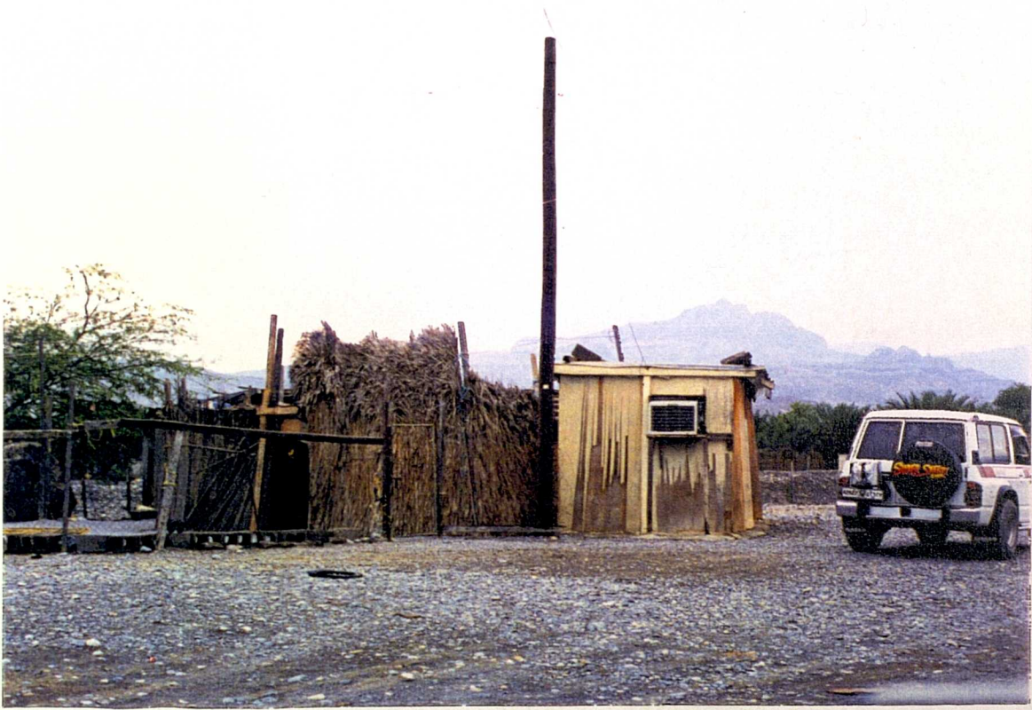
Plates 5.17. and 5.18. Squatter houses built of palm leaves and plywood
