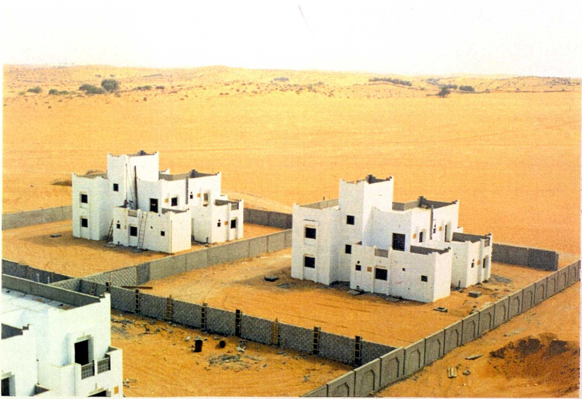
Plates 3.17. and 3.18. Low-cost houses under construction
