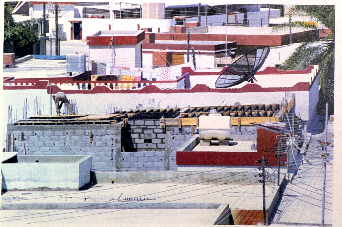
Plates 6.11. and 6.12. Private house built of popular construction
