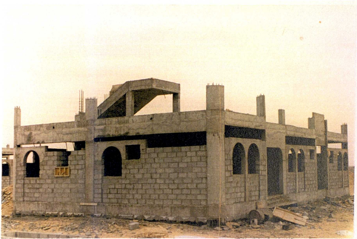
Plate 6.1. Reinforced concrete construction for single storey low-cost house
