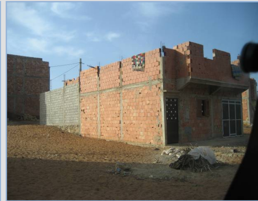
Middle and right: New construction by the bidonville residents on freshly allocated serviced plots. Most houses use perforated brick and concrete for construction, and follow the plan given to them by the developer.
