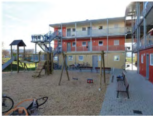
Playground / Photo: © Heiner Holme
