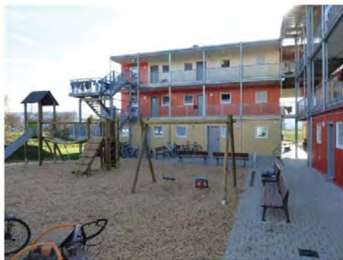
Playground / Photo: © Heiner Holme
