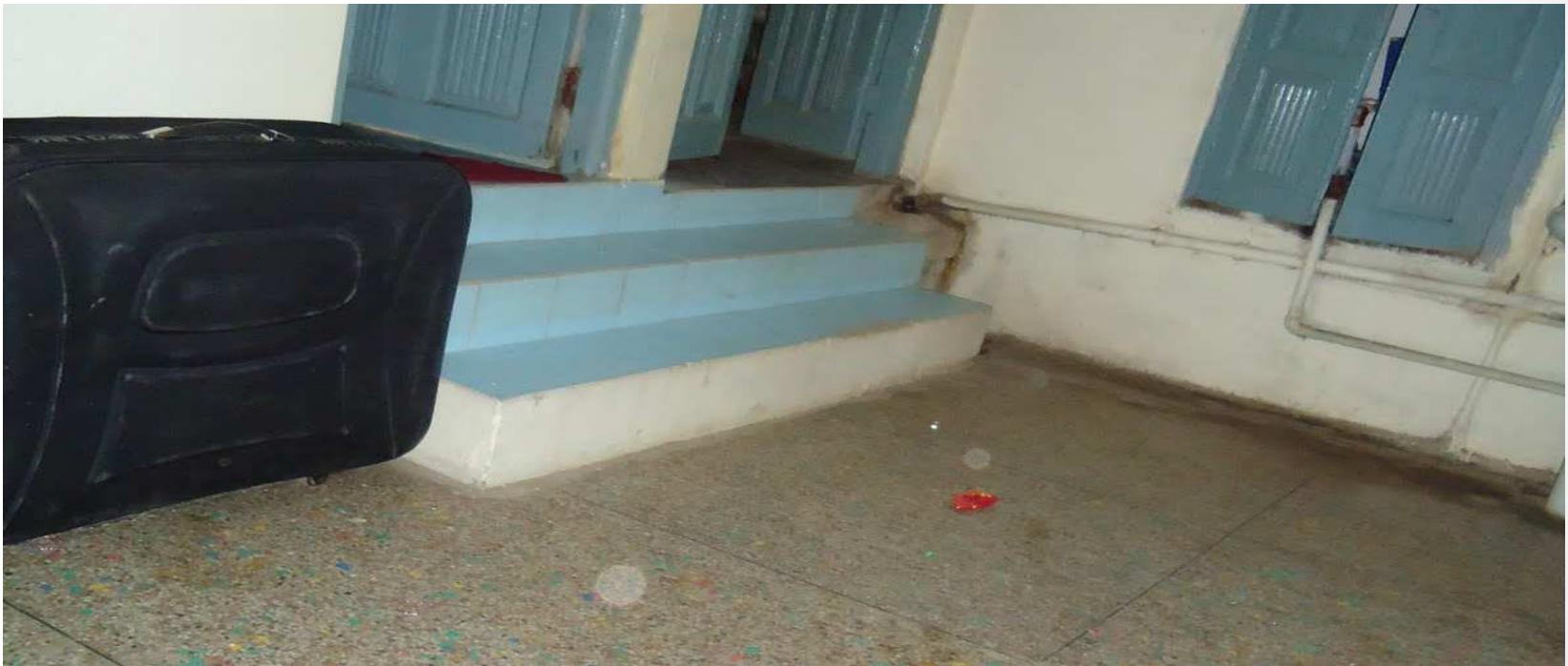
Newly constructed stairs after rise in road level
