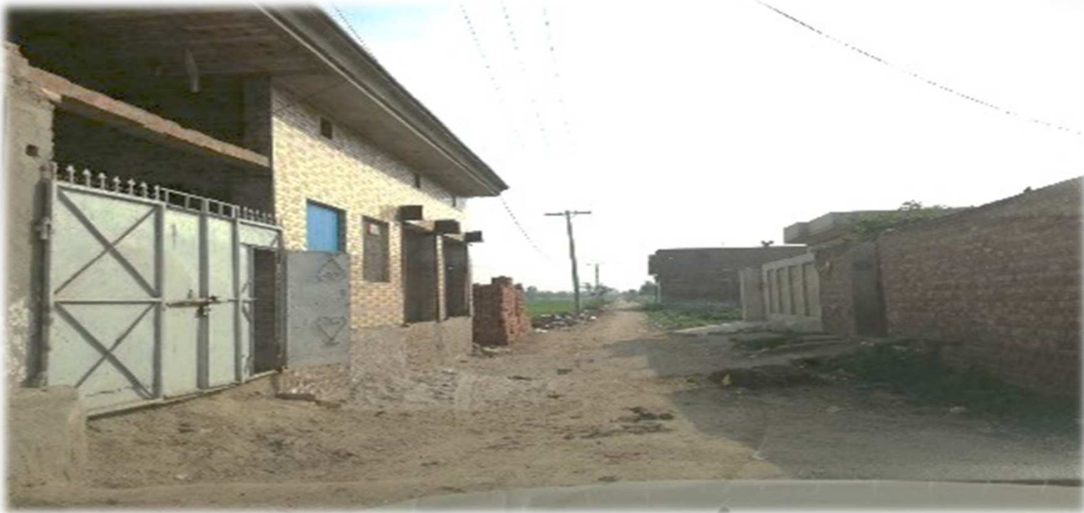
IMPROPER HOUSE FACADES
