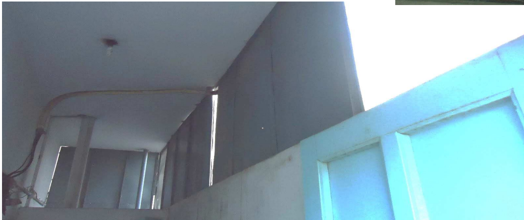
Open Shafts In bathroom
