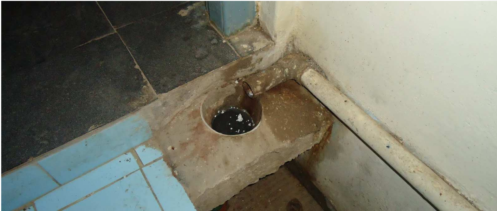
Newly constructed open drainage after rise in road level
