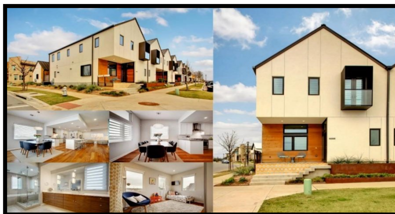
Figure 3. Tilley Row House, Austin, TX, USA. (Hsu , 2022)
