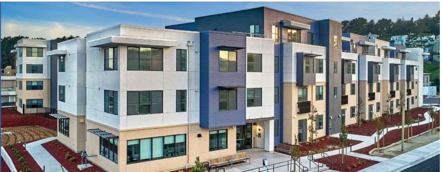
705 Serramonte school employee housing.
