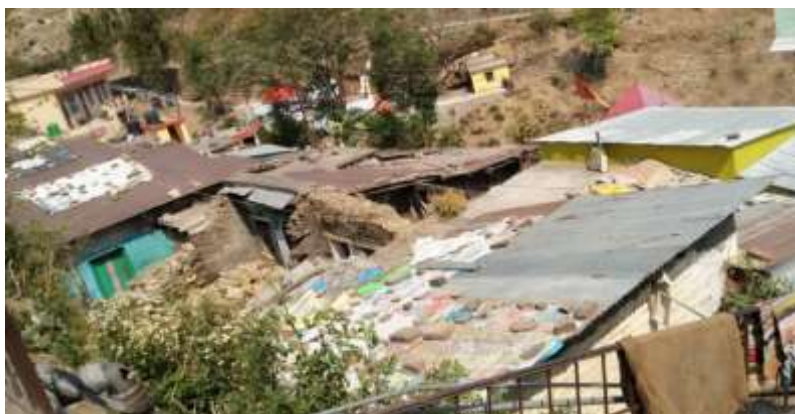
Photo Plate 1: Poor Condition of Houses
