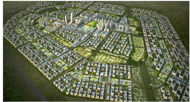
Figure 1. Aerial view of the Bismayah residential project [11]
