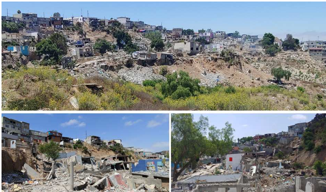
Fig. 2. Area affected by a landslide that continues to be active.
