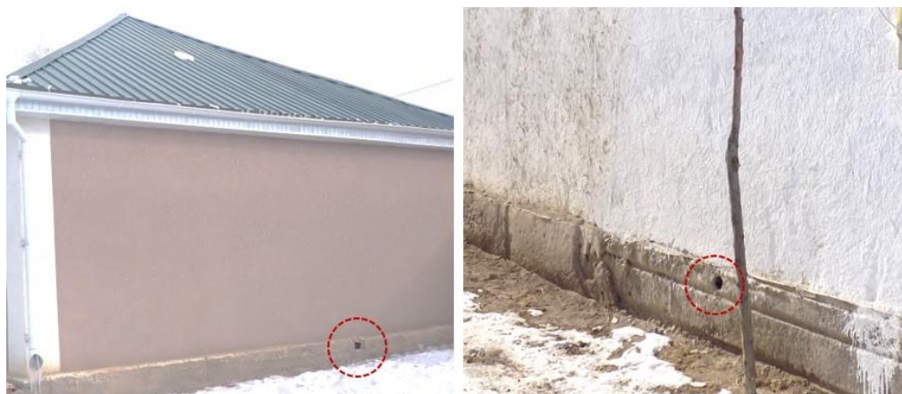
Figure 10. Natural ventilation inlet/outlet to the environment in the floor of rural Kyrgyz houses.
