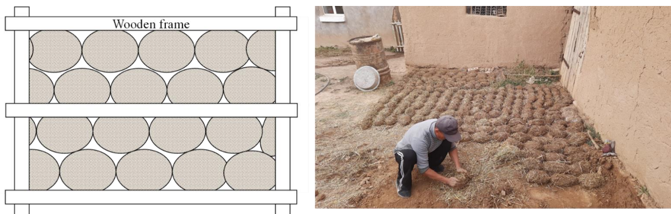
Figure 13. A wall structure with clay lumps and a wooden frame (left) and clay lumps in preparation (right).
