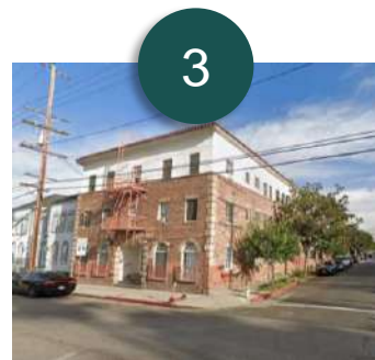
Alegria Apartments Esperanza Community Housing Corporation
