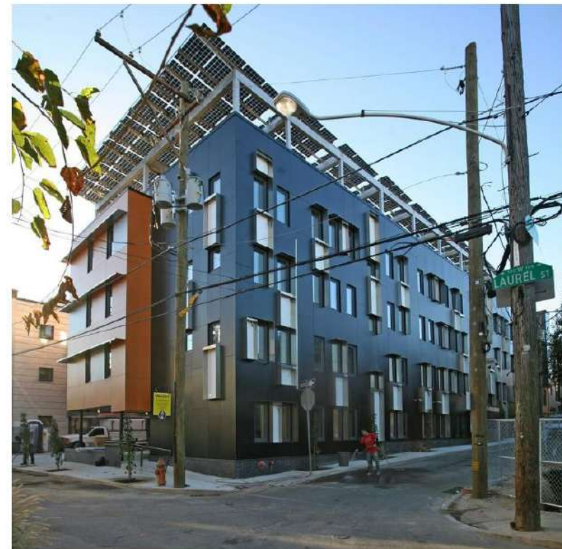
Phase III of the Battery, Philadelphia, PA – New Market Rate All Electric Housing with Rooftop Solar PV Source: onionflats.com
