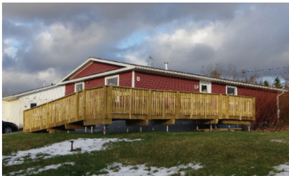
A public housing three-bedroom home adapted to be accessible for a Cape Breton family.
