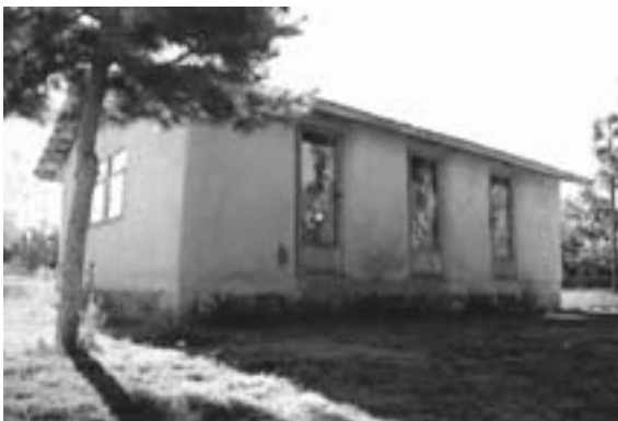
Fig. 7. The straw-bale building in Hasandede, Kırıkkale (photograph by Zeynep Arsan)
