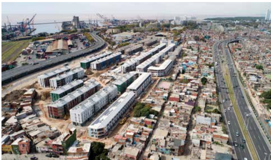
New homes currently being built in Barrio 31.
