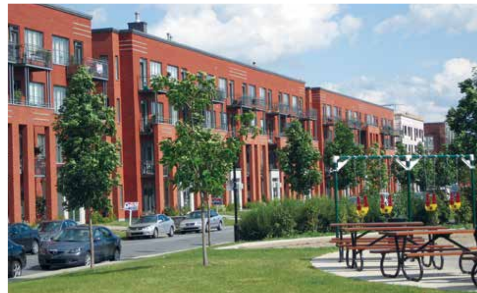
Recent condominium project—8 plex. Typical in the central districts and the surrounding boroughs. More affordable because the structure is built from wood and the design is both economical and efficient.
