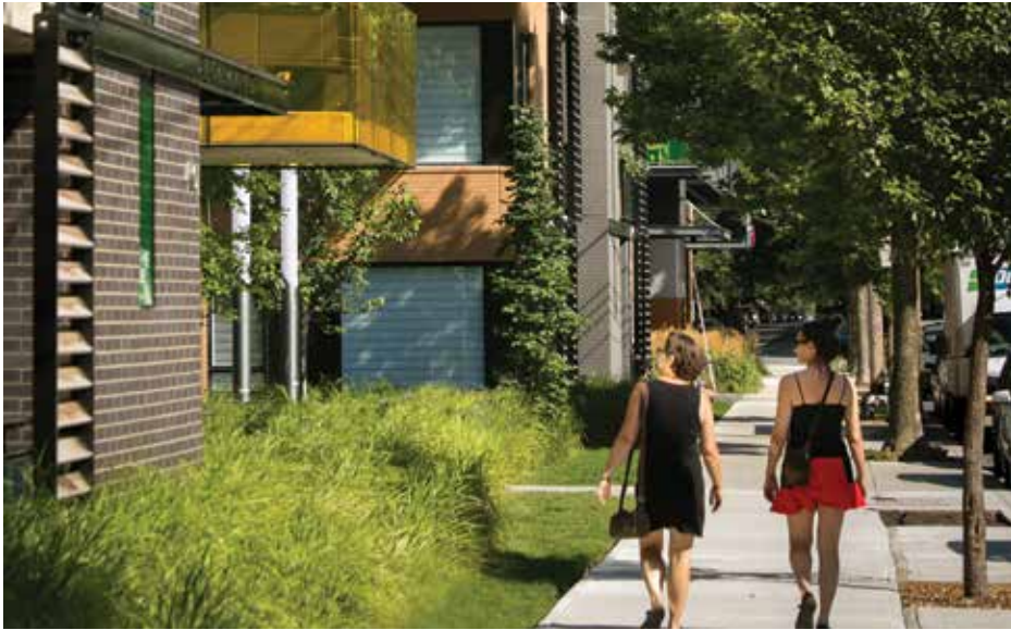
Platopolis: Inclusionary project comprised of 236 units in total, 190 private condominiums (including more than 30 % of 3 bed units) and 46 community housing units (COOP).
