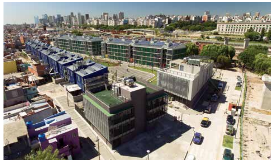
Sustainable features incorporated into the design of the new Barrio 31 homes.
