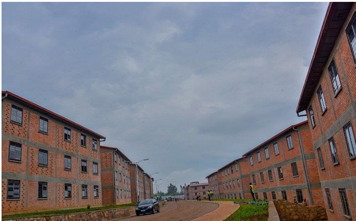
Figure 10: Busanza Housing Estate - Source: (Rwanda Housing Authority, 2024)
