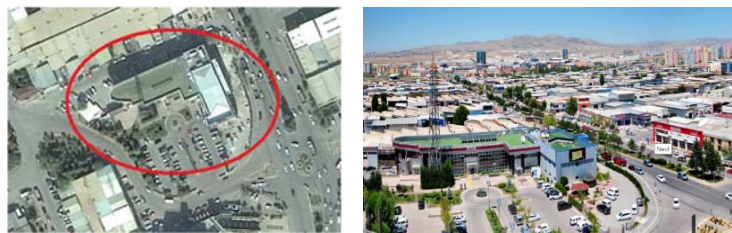
Figure 1. The satellite image and a view of OHQ Building [22, 23]
