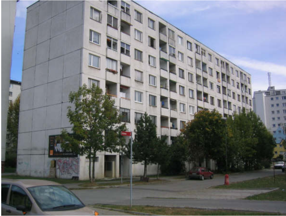
Figure 1: An image of high-rise residential buildings 'panel flats' in Martin (Habitat Platform, 2006)
