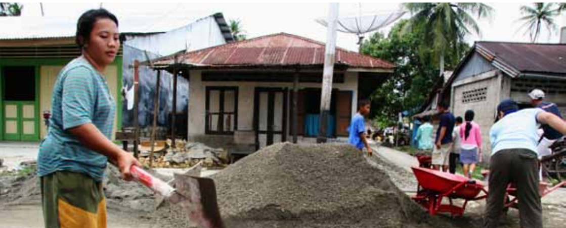
Collective self-help housing construction © UN-HABITAT
