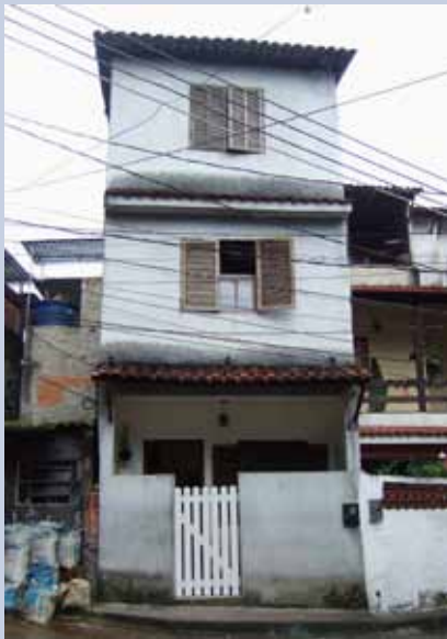
Figure 7: Incremental self-built housing in Favela Mata Machado, Rio de Janeiro, Brazil © UN-HABITAT/ Claudio Acioly
