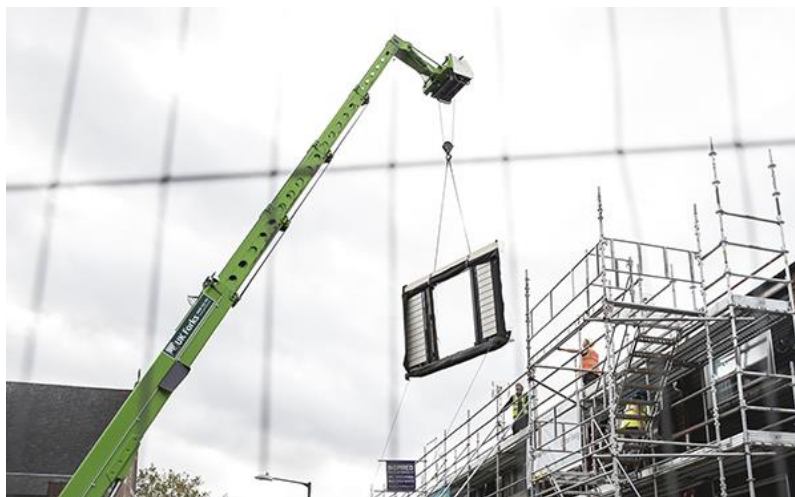
Figure 14: Installation of premanufactured facade in an Energiesprong project in the United Kingdom
