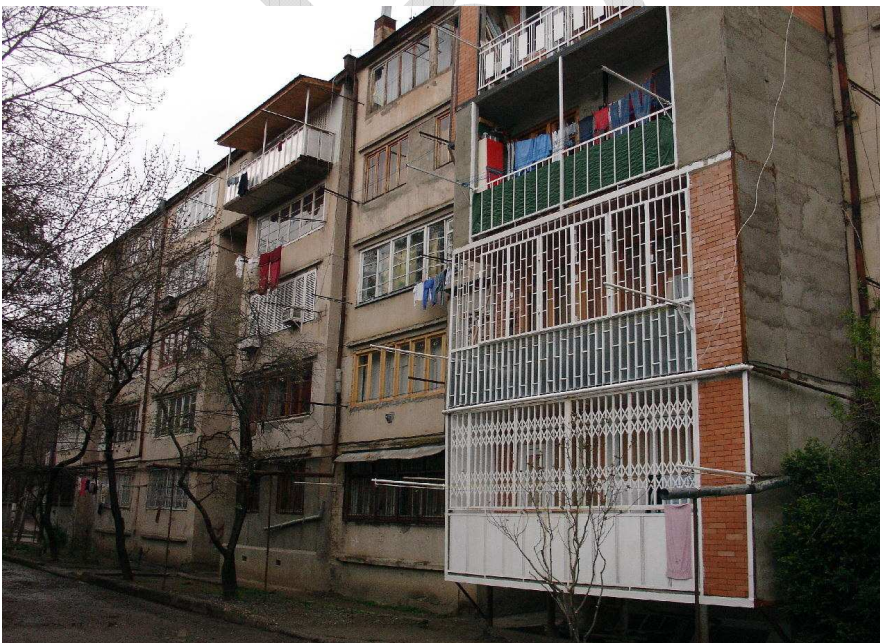
Figure 3: Deteriorating quality in privatised housing in Tbilisi
