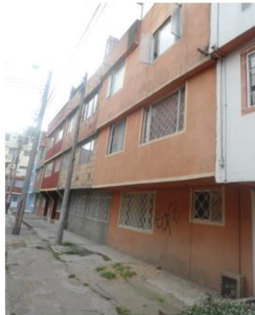
Figure 36: Row houses A1-A2: To the left: unplanned expansion onto adjacent public open space. To the right: expansion of second and upper floor's area pushing out each from the wall of lower floor
