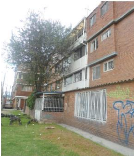
Figure 36: Row houses A1-A2: To the left: unplanned expansion onto adjacent public open space. To the right: expansion of second and upper floor's area pushing out each from the wall of lower floor
