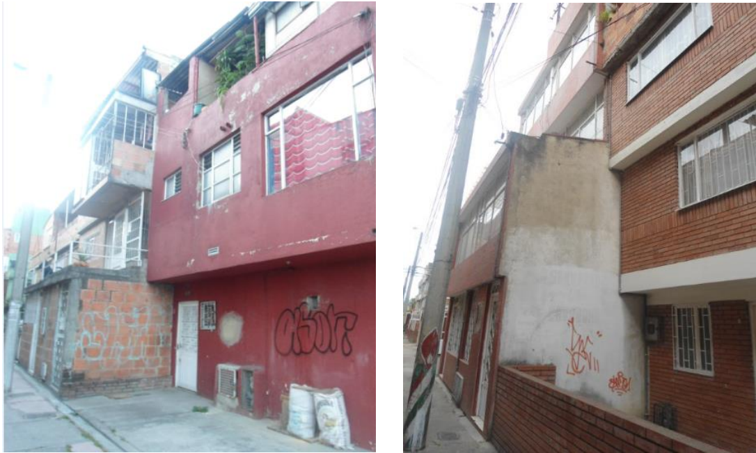
Figure 37: Row houses A1-A2: Unplanned expansions for additional rooms using the community street
