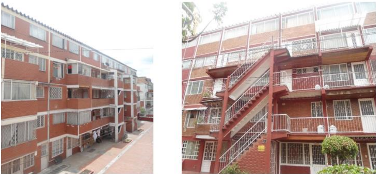
Figure 51: Examples of building façades of type D.
