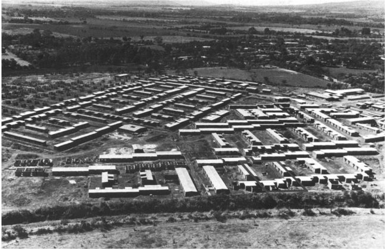
Figure 5: Aerial view during construction, c.a. 1979.
