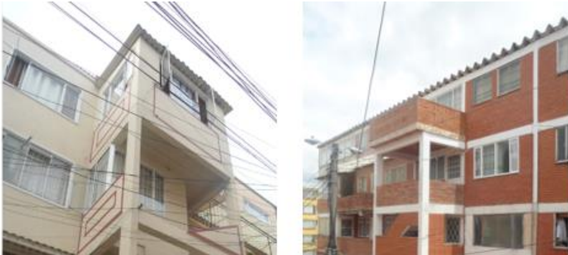
Figure 49: Examples of unplanned expansions on the community rooftop staircase.
