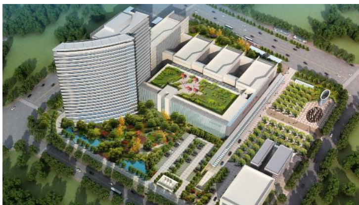
The newest Xiangtan hospital will be able to withstand severe flooding due to the presence of large run-off areas, underground storage tanks, and back-up generators in case the grid experiences a blackout (photo by Xiangtan PMO/design institute).
