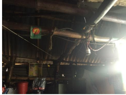
Figure-3: Condition of electricity in the area Source: Field survey, 2017
