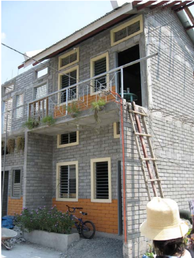
Fig. 15 Ready construction, Pasay, 2007-04-17
