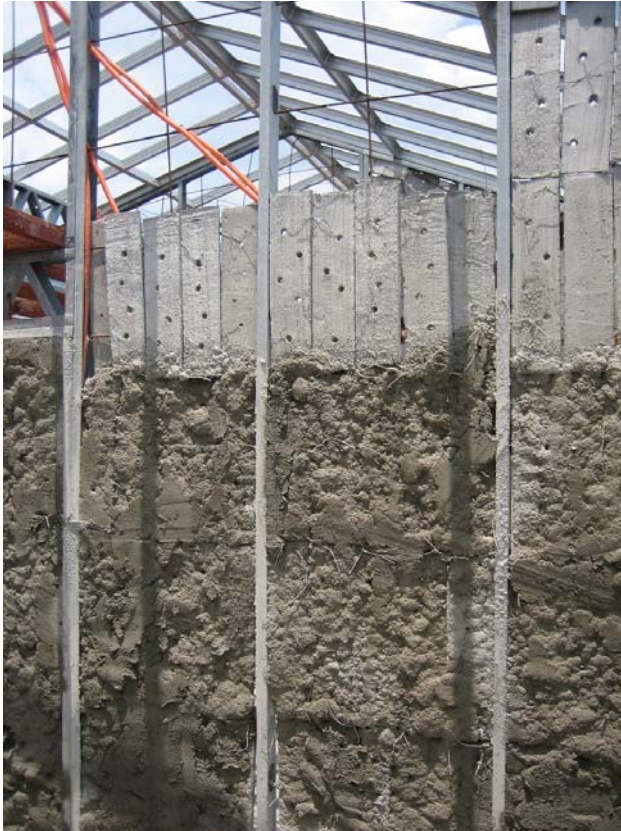
Fig. 4 The construction, Baguio, 2007-05-02
