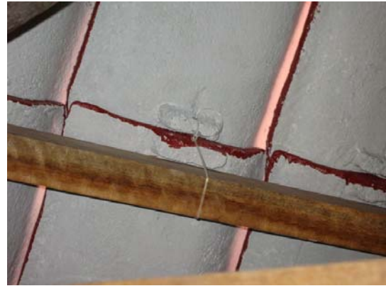
Fig. 30 Tile anchored with nylon, Sanagmana, 2007-04-14
