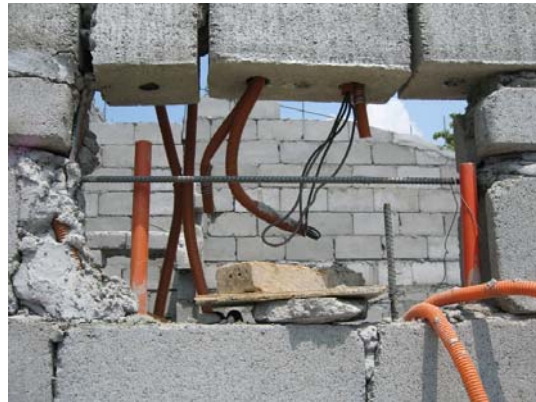
Fig. 36 Reinforcement and installation, Pasay, 2007-04-18
