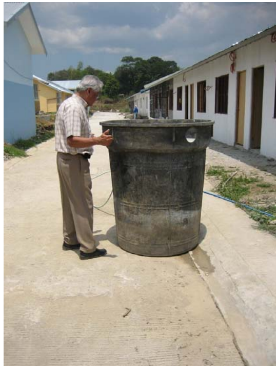
Fig. 8 The septic tank, Baguio, 2007-05-02
