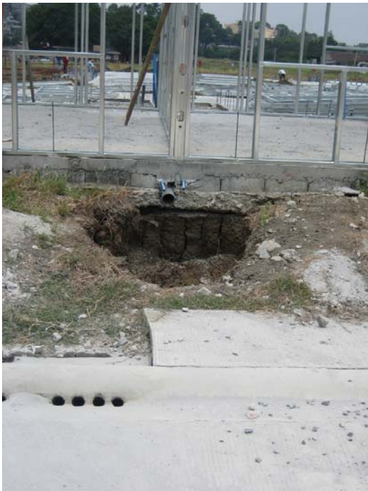
Fig. 7 Preparation for the septic tank, Baguio, 2007-05-02
