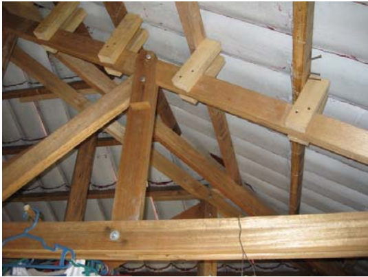
Fig. 29 Roof construction, Sanagmana, 2007-04-14
