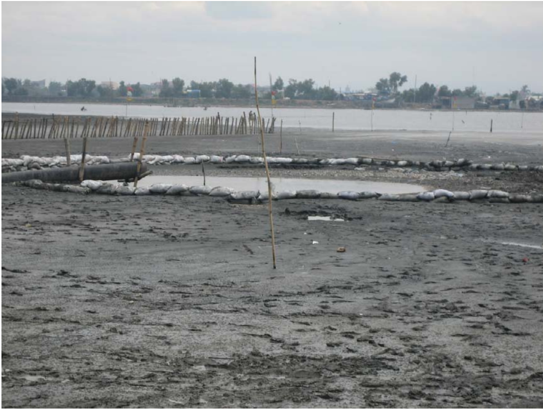
Fig. 24 Filling up the land with silt, Sanagmana, 2007-04-28
