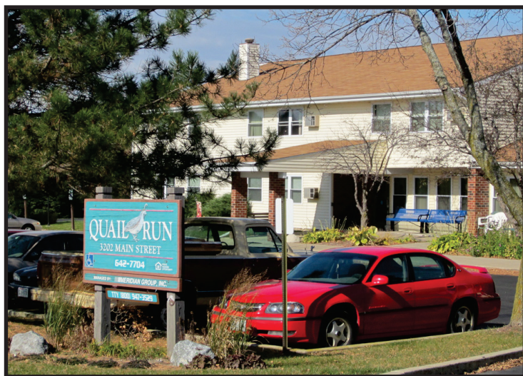
Apartment building for senior citizens and persons with disabilities in the Village of East Troy, developed with tax-exempt bonds from the Wisconsin Housing and Economic Development Authority (WHEDA) and funding from the U.S. Department of Housing and Urban Development (HUD).
