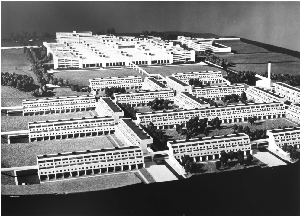
Figure 1 Southgate model photograph, illustrating the generosity of its garden squares and its relationship with the town centre
